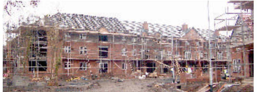
Work underway at Tarawood
