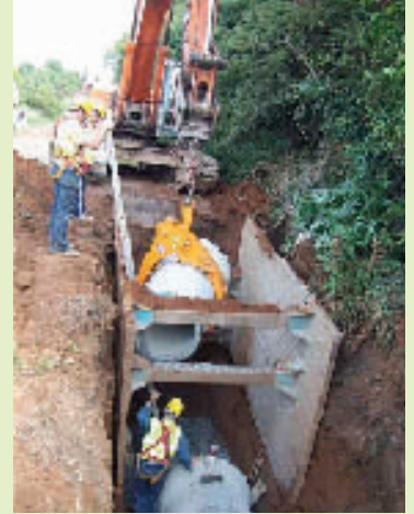
More Scott pipes are placed on a Farrans Construction site
