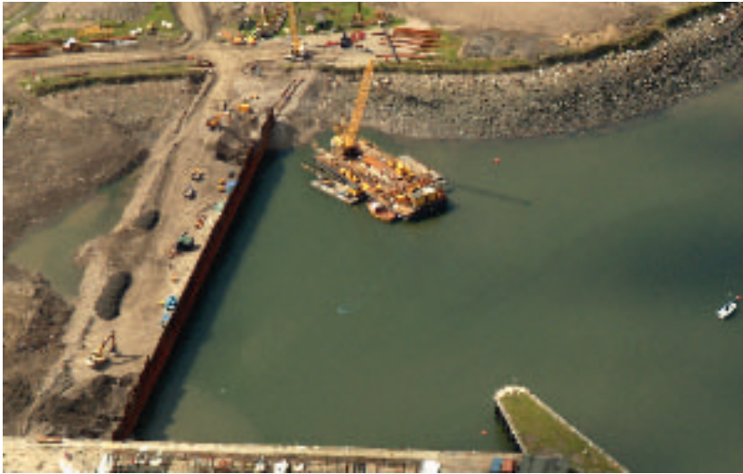
Construction work underway at Granton Harbour
