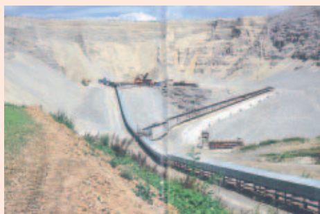
Aggregate production in a Hastag quarry at St Gallen in Switzerland
